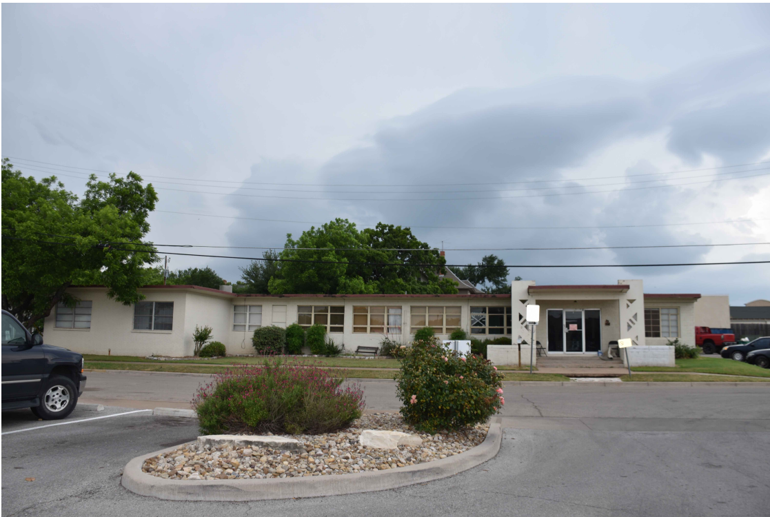
Photo 2: East elevation or front of Granbury General Hospital.
